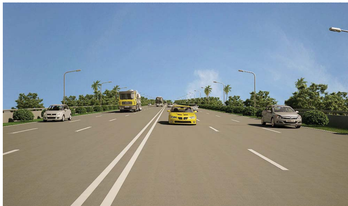
Elevated Roadway with sustainable solutions - view from roadway
