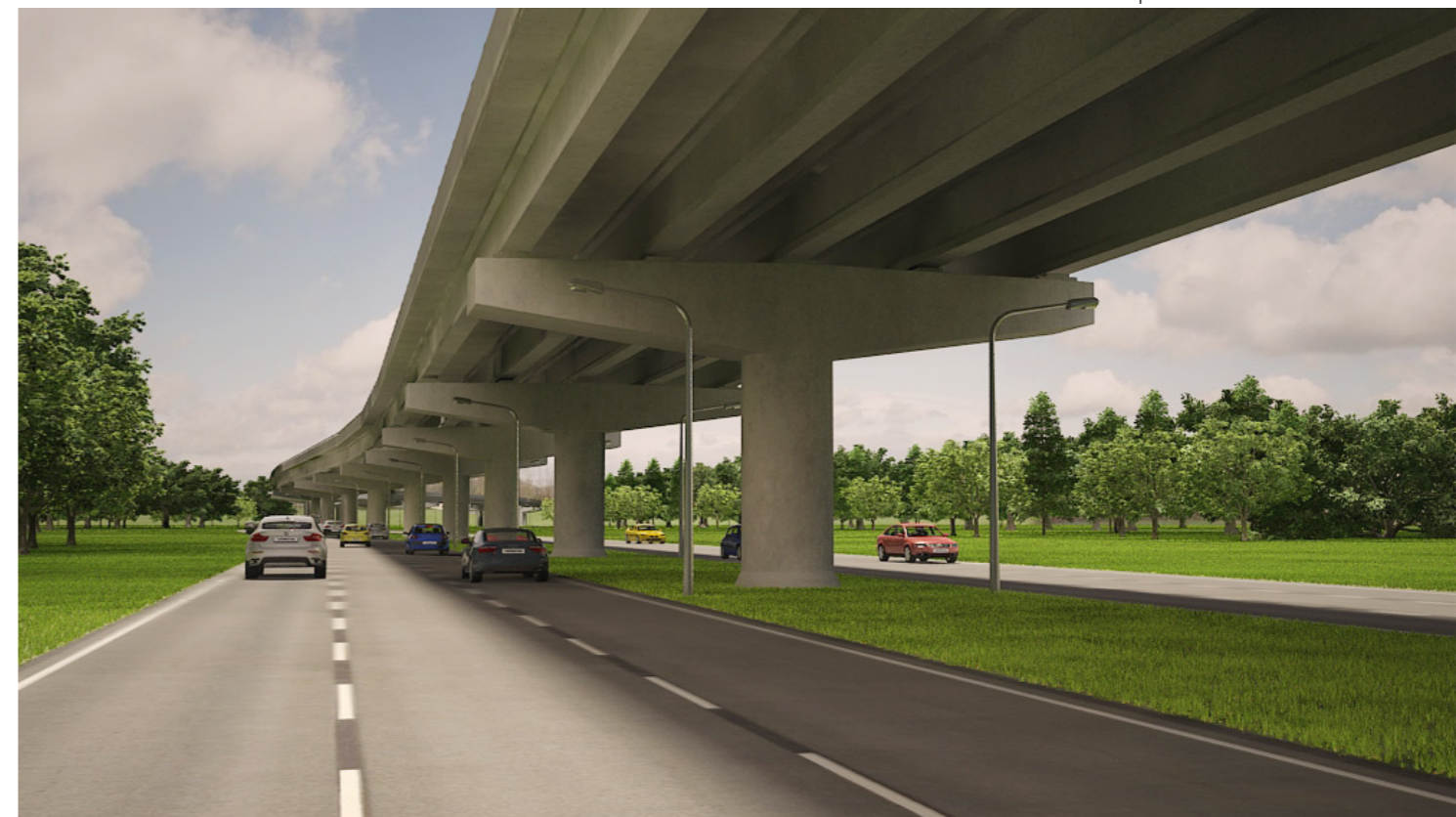
Elevated Roadway - view from underneath
